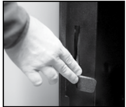
Double door handle down to unlock left door.
